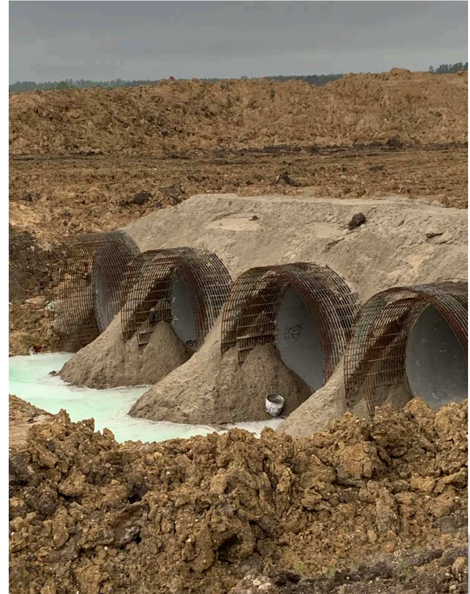
Luce Bayou Canal near Grand Parkway
