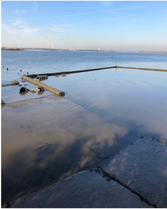
Home foundation remnants inundated
