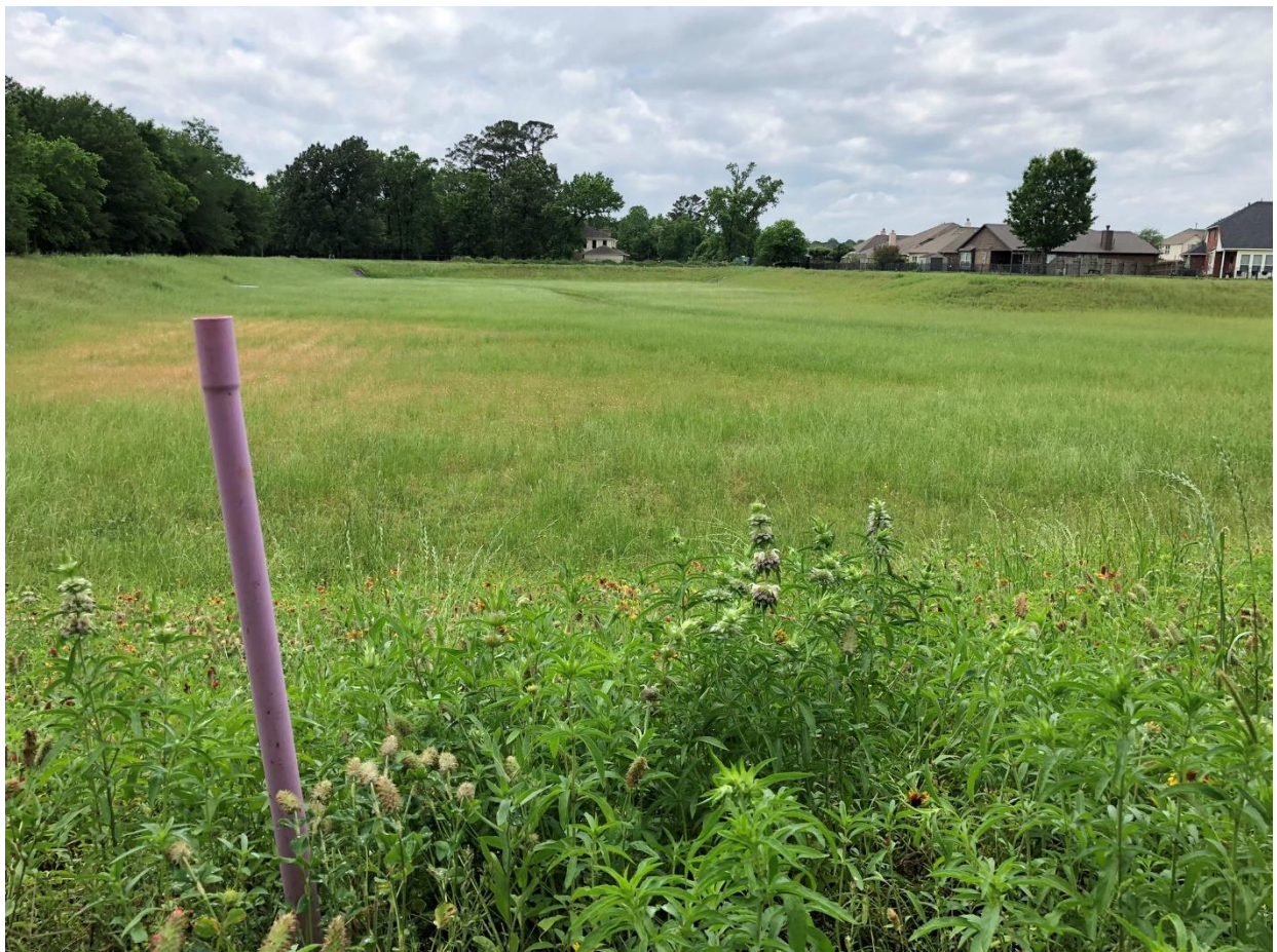
Image 4. Purple pipe coming out of the ground at detention pond to indicate to landscapers of spray heads to avoid when mowing.
