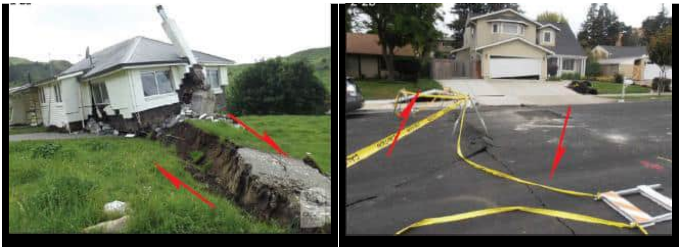
Figure 28: Impacts of surface fault on a house. The house shown on the left collapsed due to extreme damage and the house shown on the right suffered moderate damage resulting in costly repairs. Red arrows show the relative trend of horizontal movement. (CADC, CGS, 2018)
