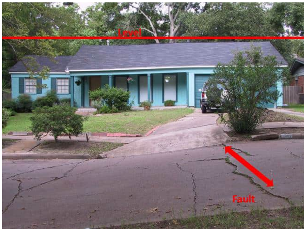
Figure 29: Impacts of Long Point surface fault on a road. ix
