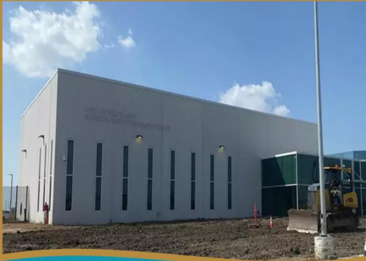
Pearland Water Treatment Plant
